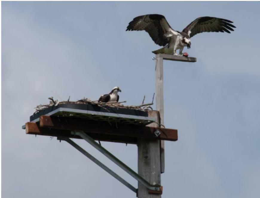
Figure 1. Osprey nest platform with offset design
