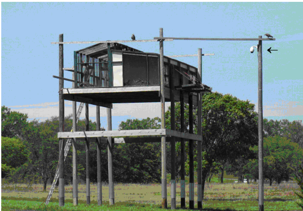
Figure B. Hack tower used at Lake Yankton, SD reintroduction site from 2008-2010. Note the drop-down doors at the upper right portion of the structure and the observation camera (indicated by arrow) mounted on the separate pole at the extreme right. Access to the rear compartment of the tower (left side of this view) allowed hack site attendants to deliver food and medical care. The ladder was used by hack site attendants and was removed after each use. Horizontal boards allowed birds to land on the structure as they learned to fly. Predator guards at the base of the support poles discouraged predators from climbing the tower.
