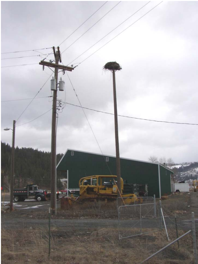
Figure 20. Poles with nest platforms can be installed to encourage osprey nesting where suitable nest structures are unavailable (a), or to coax them away from electrified poles (b).
