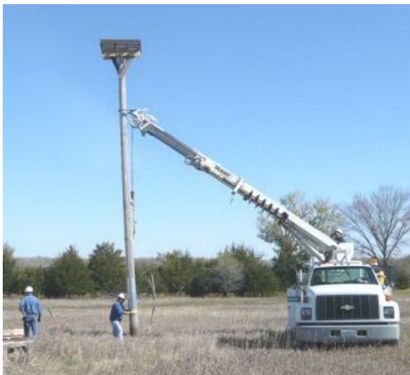
Figure 2. Nest platform installation (similar design used near site of Yankton, South Dakota area osprey reintroductions)
