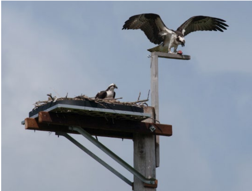
Figure 1. Osprey nest platform with offset design
