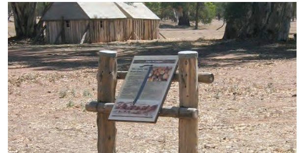
RUSTIC TIMBER & POST SIGN PANEL MOUNTING
